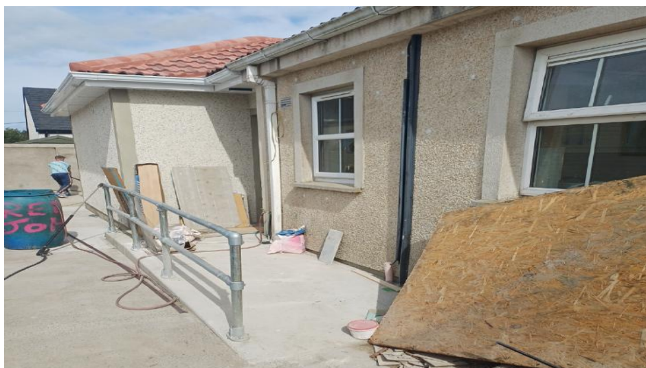
Works ongoing extension at No.7 Ballintесkin August 2026
