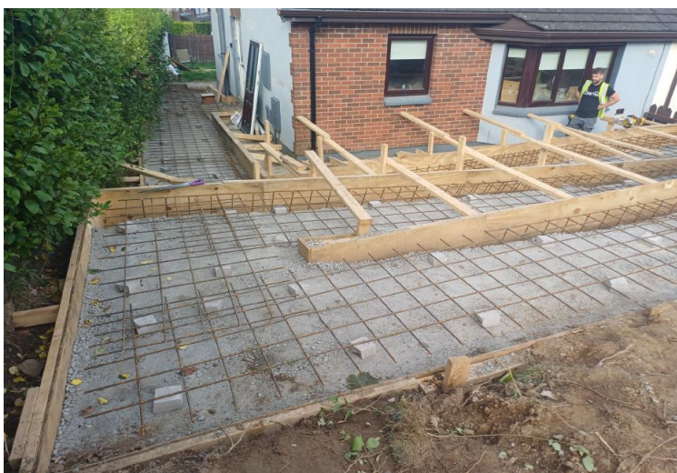
Disability Grant Works at 6 Woodbrook Arklow
