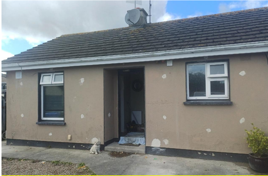
Energy Retrofit works Walls being pumped at Asgard Close Arklow Town. August 2026
