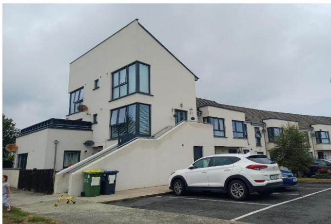
New windows and doors installed at Farrenkelly Greystones 2026
